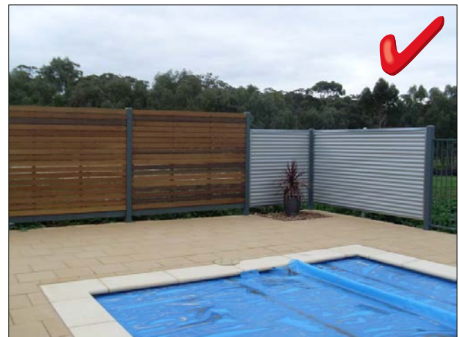
Above: example of fencing using timber, corrugated iron and traditional tubular pool fencing. Note, no gaps greater than 10mm between the sections of timber and no gap greater than 100mm below the fence.
