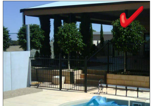
Above: example of fencing combination using blue board and tubular fencing styles. Note the fence over the retaining wall step to ensure the minimum height is maintained.
